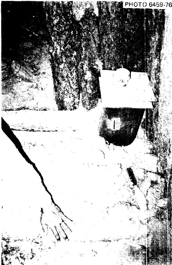
Fig. 4.9. "Puffed-up" part of the floor of Small-Pole Shelter due to the start of earth flow under moderately long-duration blast overpressure at the 53-psi overpressure range.
